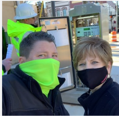
Completed Traffic Light and Curb return Project.
