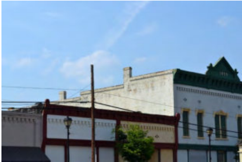
Figure 98: Parapet chimneys in the Commercial Sub-District
