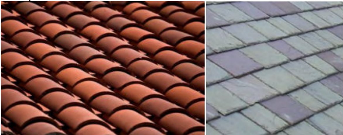
Figure 158: Clay tile shingles (left) and slate shingles (right) should only be used where they historically existed
