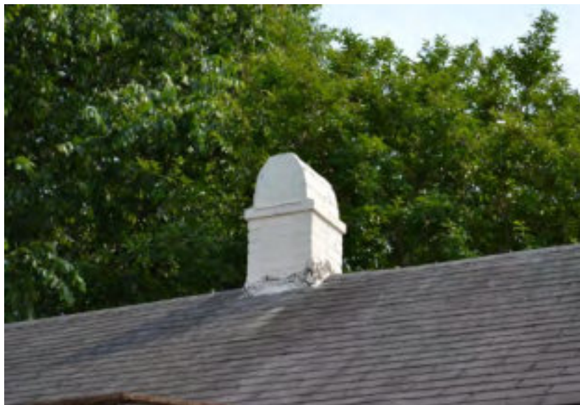
Figure 99: Chimney in a detached building in the Commercial Sub-District
