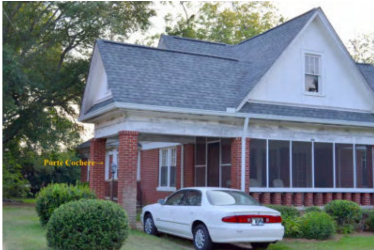
Figure 52: An intact porte cochere in the Residential Sub-District
