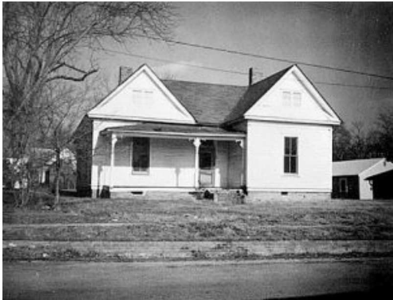
Figure 15: The Hunt family home in the Avenues and Side Streets section (photo circa 1973)
