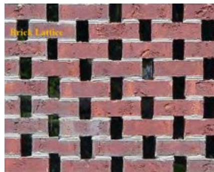
Figure 32: Brick lattice may be appropriate for replacing concrete block infill
