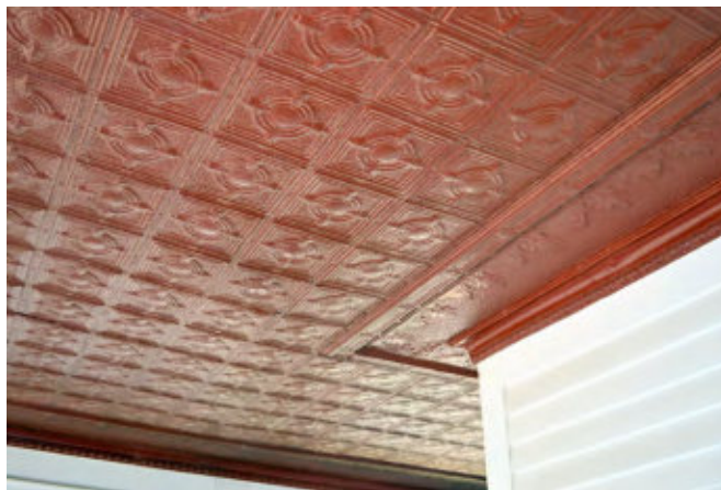
Figure 36: A rare example of a tin porch ceiling in the Residential Sub-District
