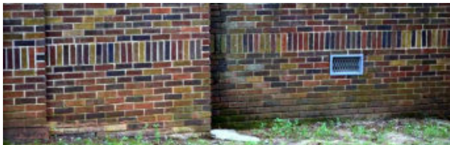
Figure 33: A continuous brick veneer foundation in the Residential Sub-District
