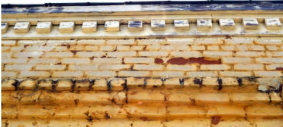
Figure 146: Parapet with a decorative cornice in the Industrial Sub-District
