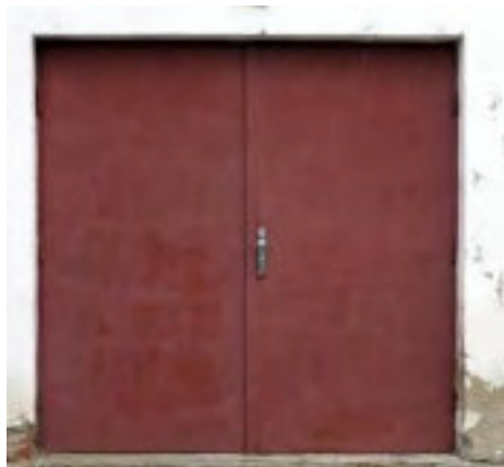
Figure 138: An acceptable replacement freight door
