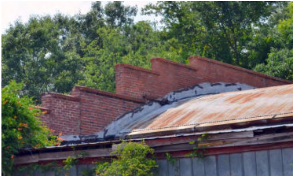
Figure 147: A stepped parapet on a warehouse in the Industrial Sub-District
