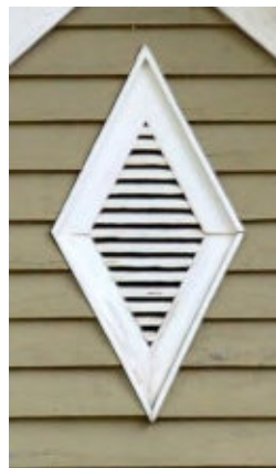
Figure 50: A nice attic vent in the Residential Sub-District
