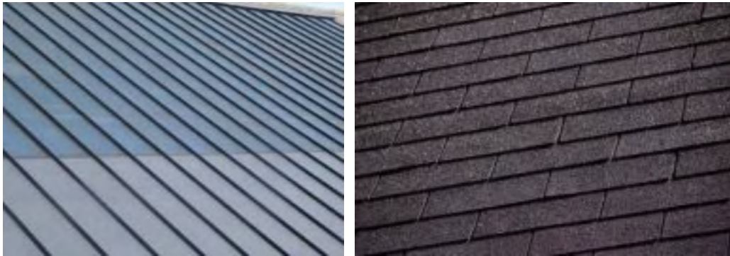
Figure 157: Standing seam metal roofs (left) and asphalt shingle roofs are acceptable for most pitched roofs
