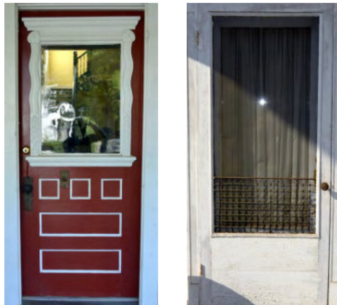
Figure 38: Some historic doors in the Residential Sub-District
