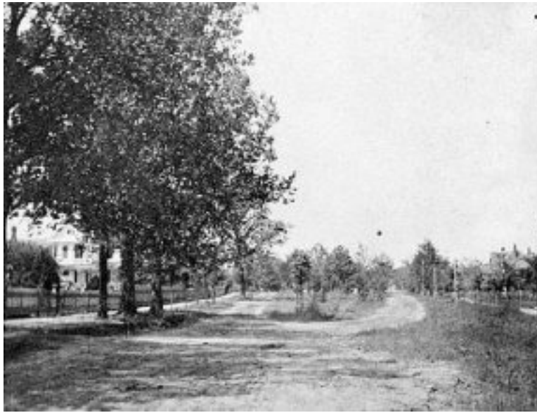
Figure 5: Looking east down East Hightower Trail in Area I of the Main Axis in 1898
