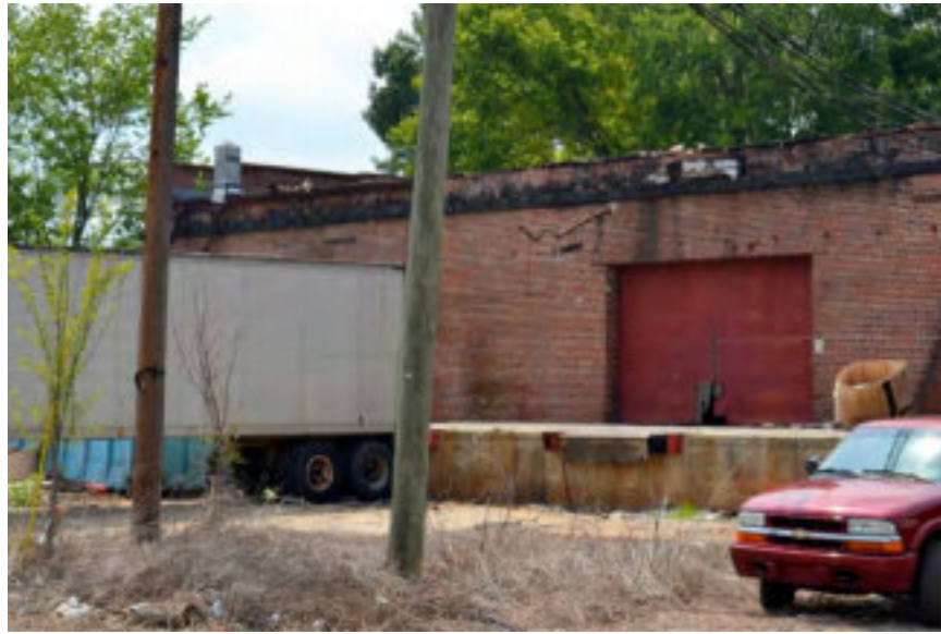
Figure 144: A loading dock in the Industrial Sub-District
