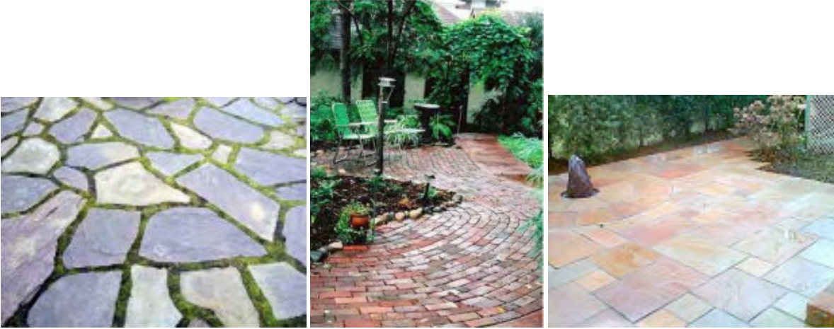
Figure 71: Some appropriate patio materials: flagstone (L), brick (M) and stone slab (R)
