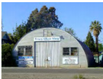
Figure 149: Quonset hut type buildings may be acceptable in some areas of the Industrial Sub-District
