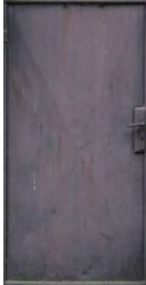
Figure 135: An acceptable standard metal door from another historic area
