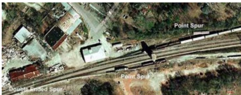
Figure 129: Some double ended and point spurs in the Industrial Sub-District.
