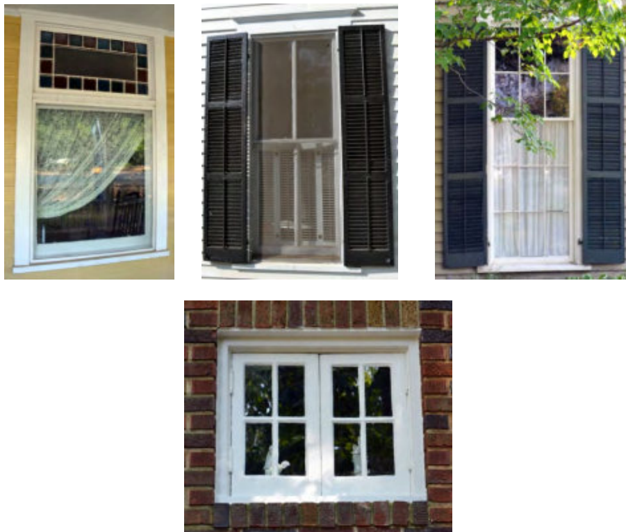
Figure 42: Historic windows and shutters found in the Residential Sub-District
