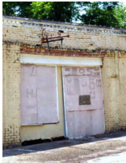
Figure 134: Patching doors with materials that do not blend in with the door itself is not appropriate
