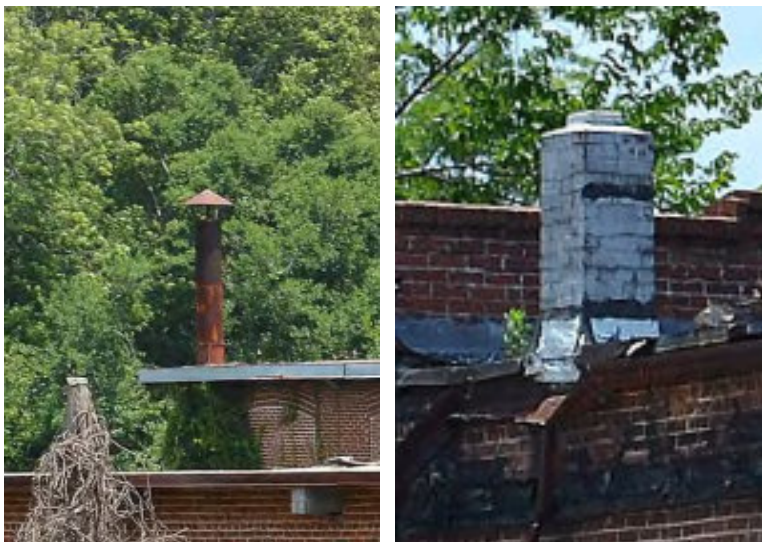
Figure 142: A historic metal smokestack and a historic brick chimney in the Industrial Sub-District
