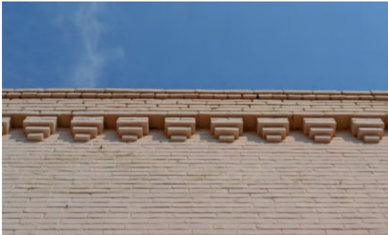
Figure 97: Parapet with a decorative cornice in the Commercial Sub-District
