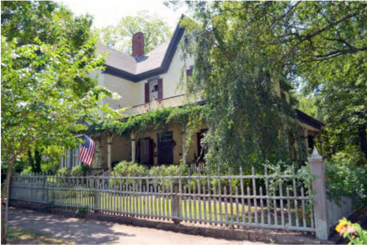
Figure 2: Robinson-McDowell-Hollis House in the Residential Sub-District
