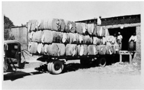
Figure 124: A cotton warehouse in the Industrial Sub-District circa 1948
