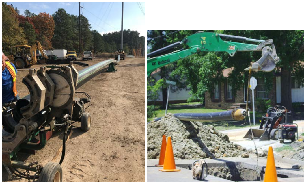
Joining Pipe and Entry Pit for Pipe Bursting (Turnipseed Projects)
