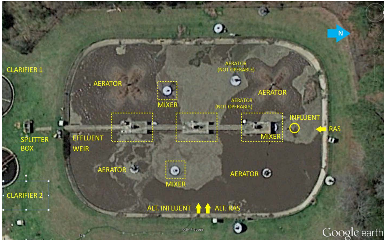
Figure 14 - Existing Aeration Basin
